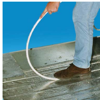
Pressing down of the heating pipes
