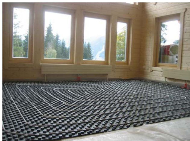
Heating for floor with nap plate system components
